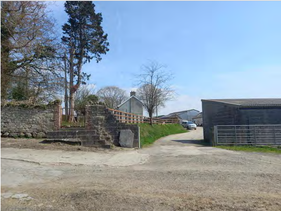
Figure 4. Hardstanding around the farmyard in poor condition with loose gravel and hard packed dirt.
