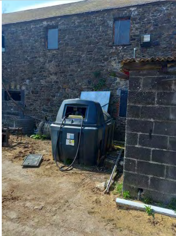
Figure 5. Oil store within the farmyard not situated on hardstanding.
