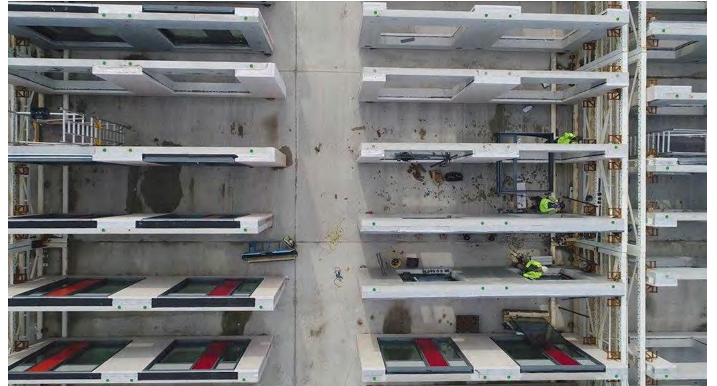
Concrete Sandwich Panel ready for assembly at Grange University Hospital
