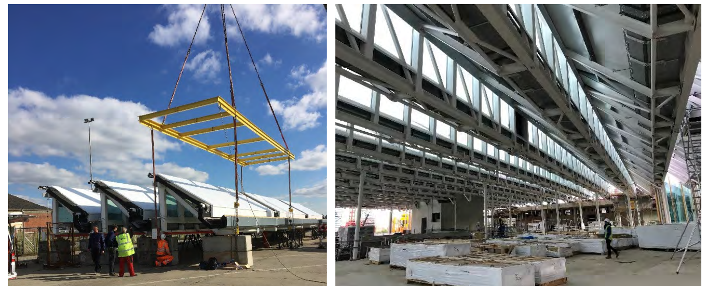
Prefabricated steel trusses complete with roof finish and clerestory glazing for AstraZeneca
